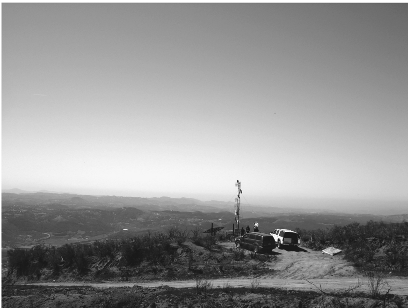
Figure 8.1 The TDV services the Adams Drive backbone tower. (2008)
